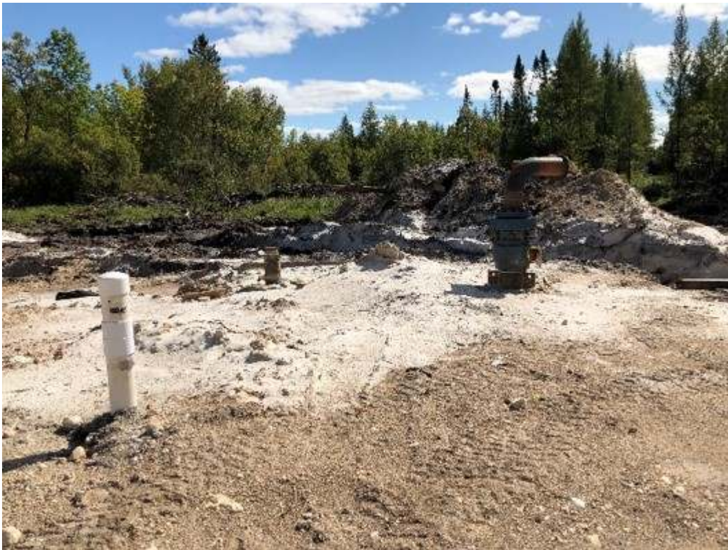
Figure 17. Unsealed CanWhite boreholes near Vivian spring, 2020.
