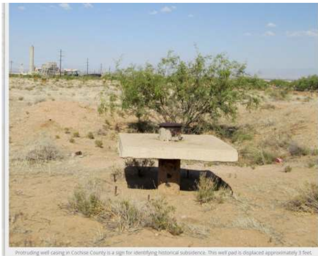
Figure 16. Land subsidence caused by declining groundwater from over pumping, exposing a borehole in Willcox Basin Arizona. Pumping from the borehole has created its own unsealed drain hole. Imagine hundreds of these boreholes filled with water from septic fields and manure following heavy rains draining into the carbonate and sandstone aquifers.
